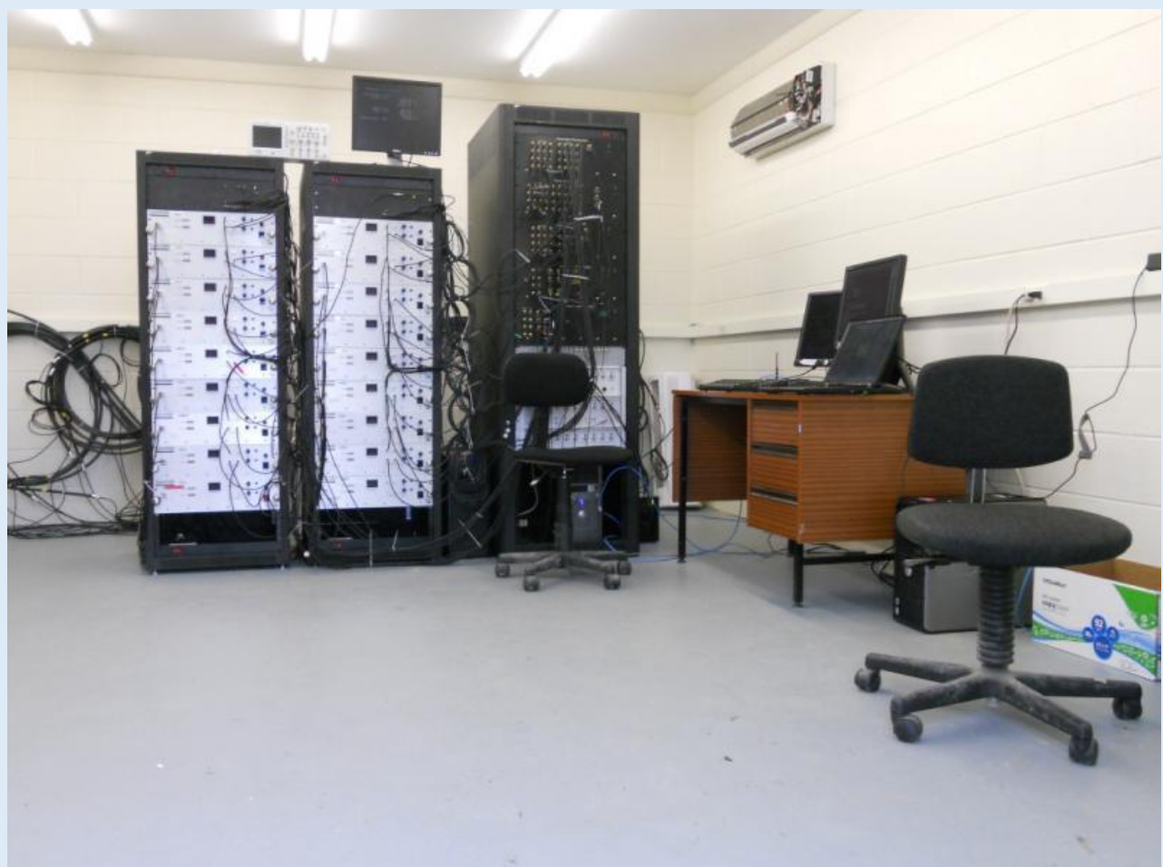
Figure 2: Image of the transmitters and computer at the Blackstone, VA site. Source: http://vt.superdarn.org/gallery
